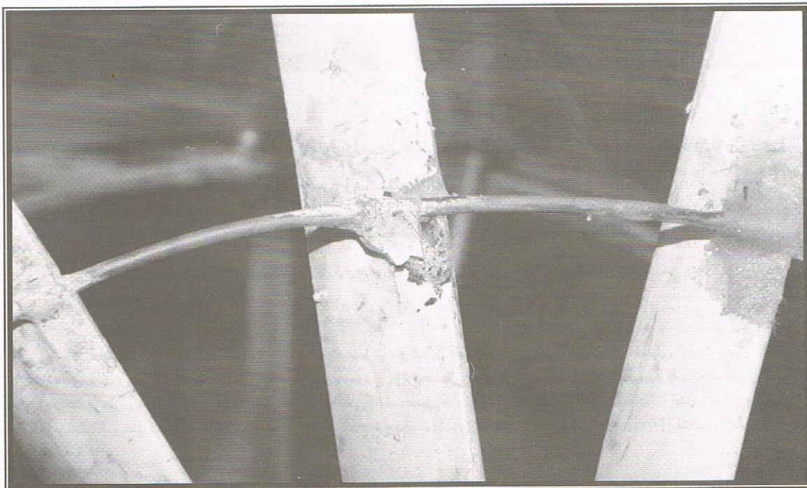
Figure (12) Failure of wind turbine in bonded joint.
