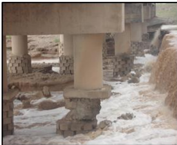
Figure 1: Damages at the Heads of Piles (Joint) and at Aspects After a site visit by the consultants team to the site of the bridge and in order to
