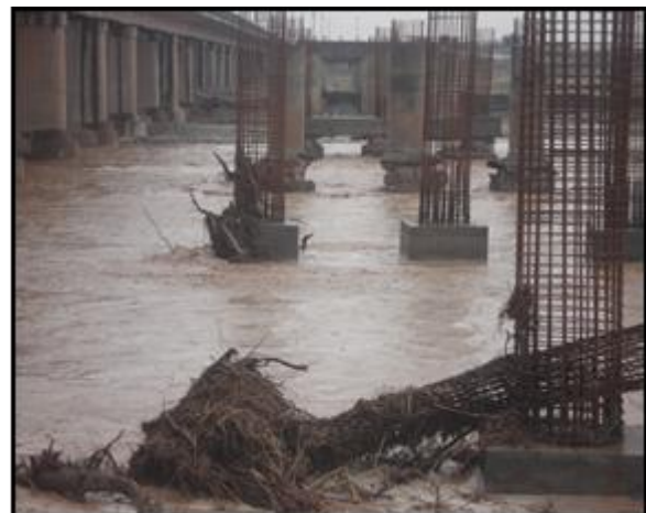
Figure 1: Damages at the Heads of Piles (Joint) and at Aspects After a site visit by the consultants team to the site of the bridge and in order to
