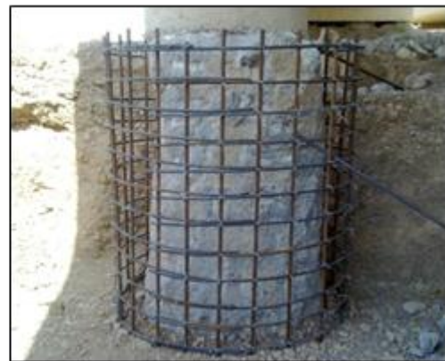
Figure 4: Installation of Steel Mesh and Steel Casing (Before Concrete Poured)
