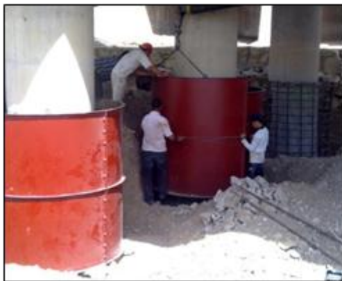
Figure 4: Installation of Steel Mesh and Steel Casing (Before Concrete Poured)
